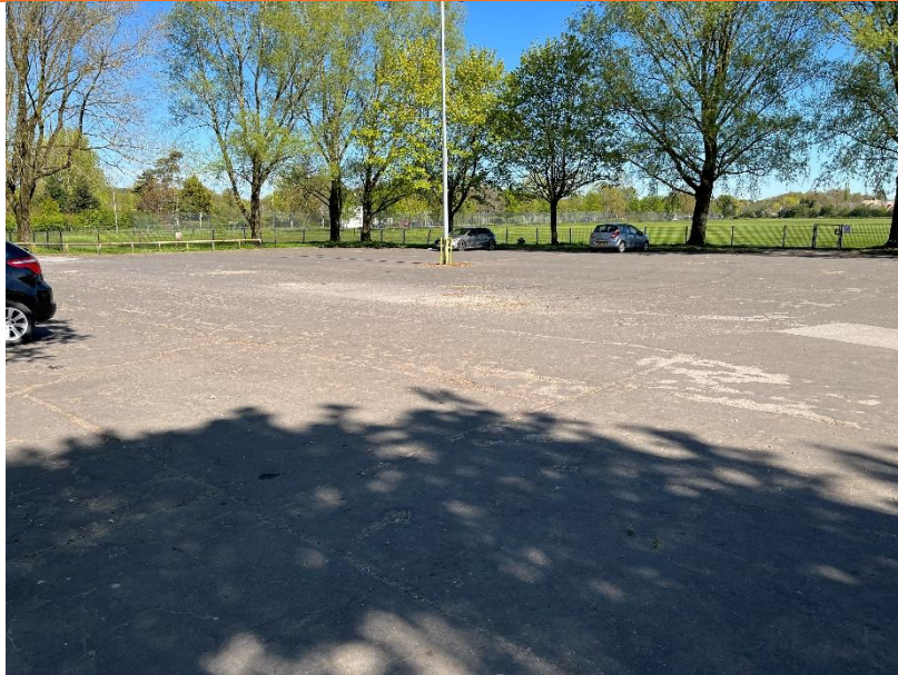
Figure 3.9 Showing Developed Land; Sealed Surface
