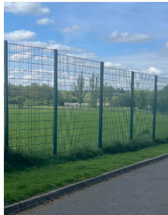
FENCE TYPE F- 3.0m Weldmesh fencing
