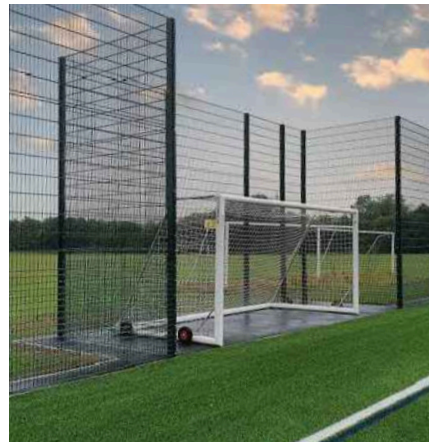
FENCE TYPE C- 4.5m Weldmesh perimeter fence
