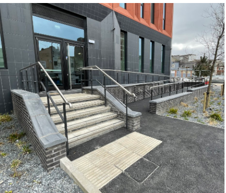
Handrails and tactile used at steps
