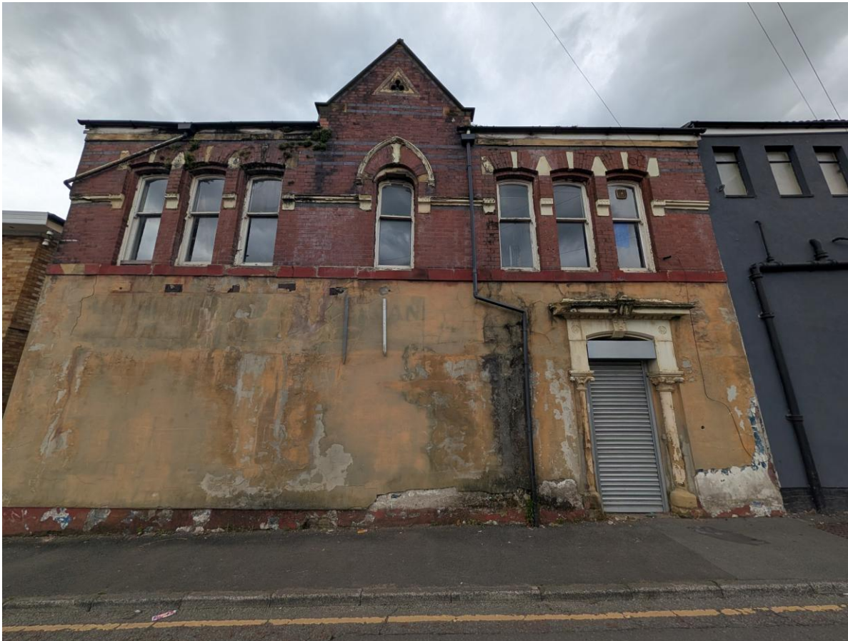
Figure 3: Existing Bethel Street elevation, with the attached neighbouring asset visible to the right.
