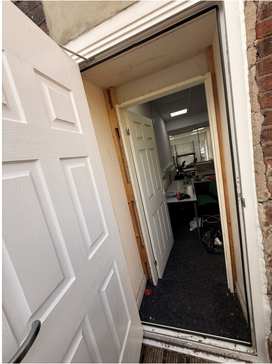
Figure 13: Existing rear exit viewed externally, showing the retained doorway and internal circulation beyond.
