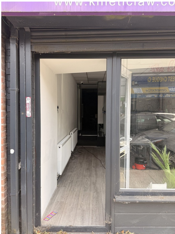
Figure 5: Existing principal entrance viewed externally, showing the retained entrance and internal circulation beyond.
