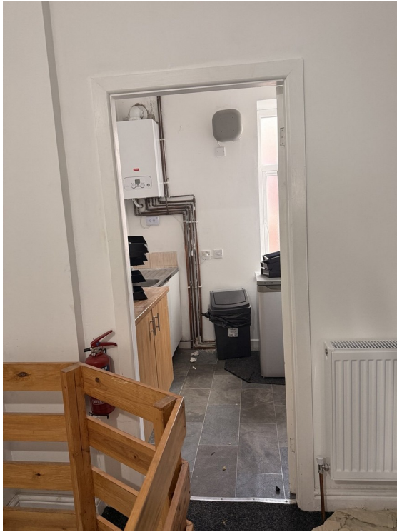
Figure 11: Existing doorway adjacent to the stair landing serving the kitchen/boiler area, identified as a location for a proposed fire-resistant door.
