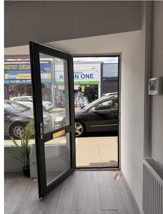
Figure 4: Existing principal entrance viewed internally, showing the retained entrance door and entrance circulation area.
