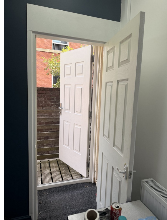
Figure 12: Existing rear exit viewed internally, showing the existing doorway and access to the rear of 146 Yorkshire Street.
