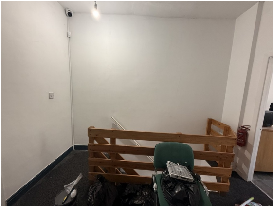
Figure 10: Existing upper landing and open timber balustrade, showing the area proposed to be enclosed as part of the fire-safety works.
