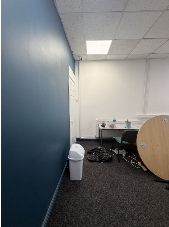
Figure 7: Alternative view of the existing ground-floor area proposed for the protected corridor, showing the current internal finishes and relationship with the existing doorway.
