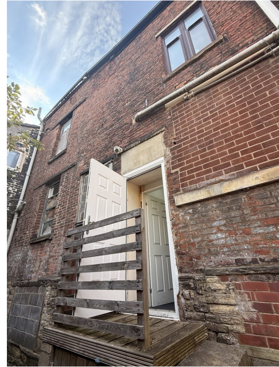
Figure 14: Existing rear elevation of 146 Yorkshire Street, showing brickwork, window openings, rear exit and associated access platform.
