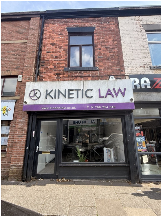
Figure 1: Existing principal elevation of 146 Yorkshire Street, showing the ground-floor commercial frontage, existing Kinetic Law fascia signage and upper-floor brick elevation.
