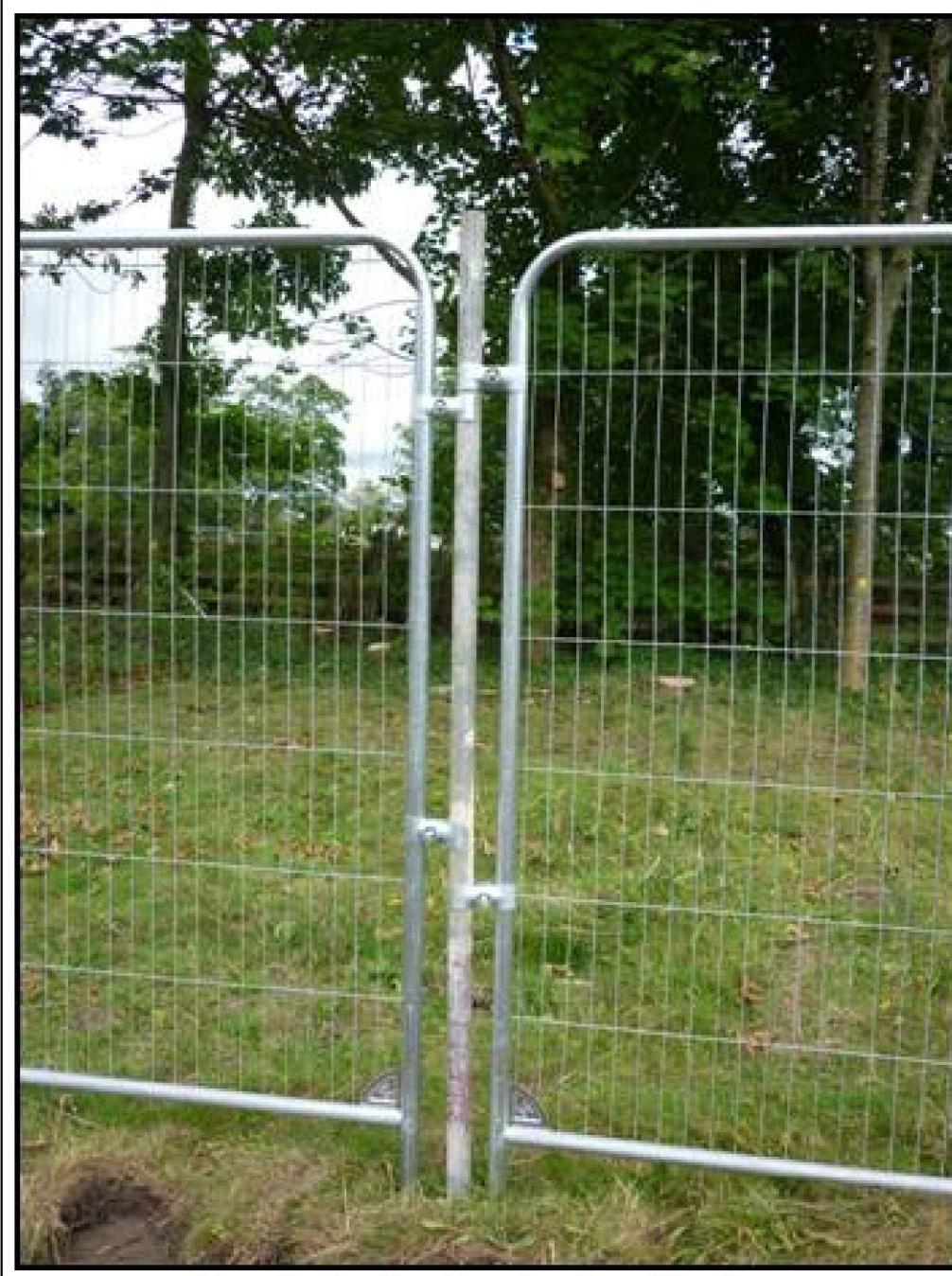
Tree Protective Fencing Specification
