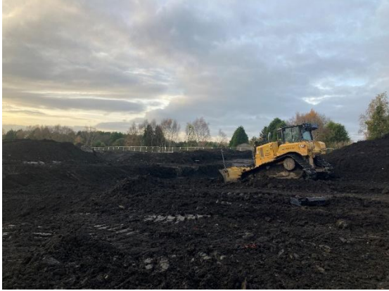
Plate 25 Replacement of Made Ground
