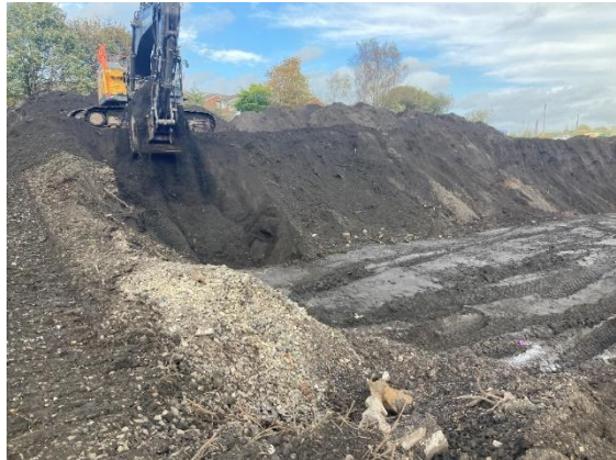
Plate 18 Made Ground Turnover
