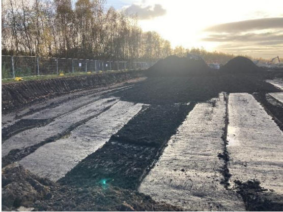
Plate 21 Placement of Final Layer (Formation)
