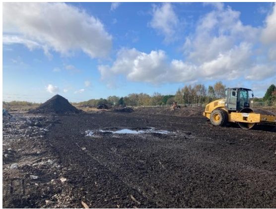
Plate 24 Placement of Made Ground
