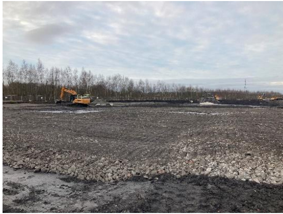
Plate 24 Placement of Made Ground
