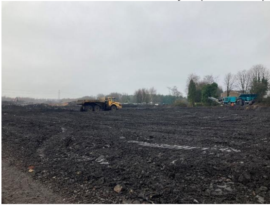
Plate 23 Placement of Pile Mat
