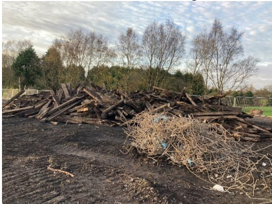
Plate 5 Stockpile Containing Visible ACM Fragments Awaiting Handpicking
