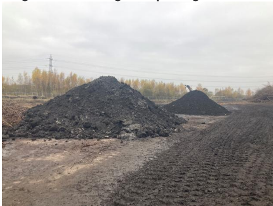
Plate 5 Stockpile Containing Visible ACM Fragments Awaiting Handpicking
