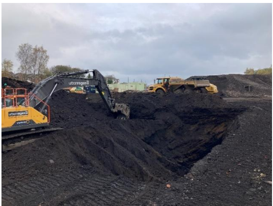
Plate 17 Made Ground Turnover
