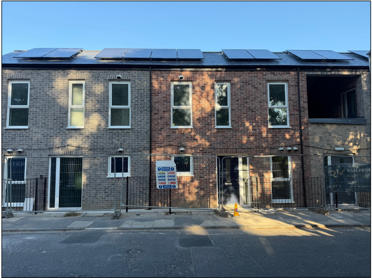
Photograph 1: Front Elevation of the site at Hornby Street in Heywood
