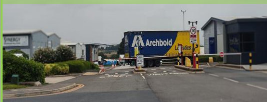
A manned gatehouse and automated vehicle barriers secure the entrance to Birch Business Park
