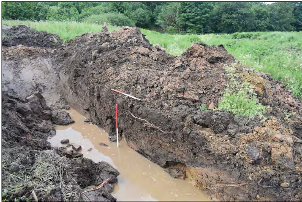
Plate 14. Southeast end of Trench 29, looking south
