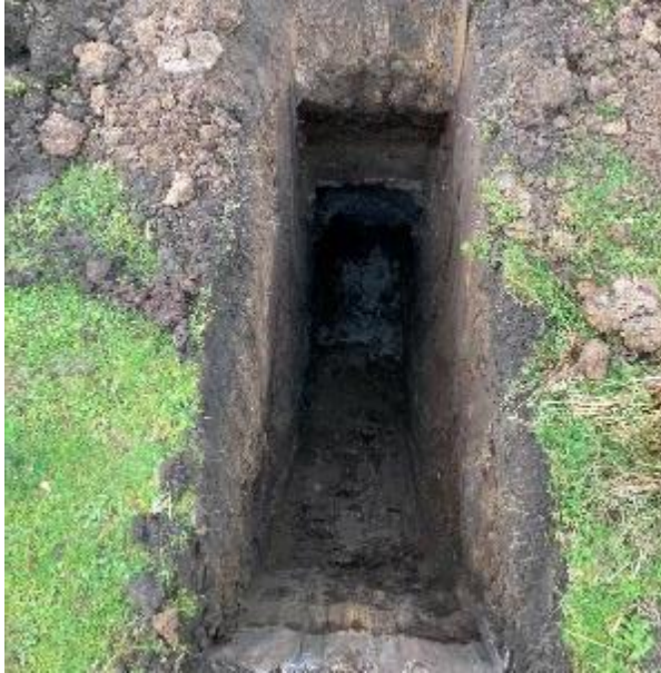
PLATE 9 TP115 EXCAVATION AND ARISINGS – NATURAL DRIFT WITH POCKETS OF PEAT
