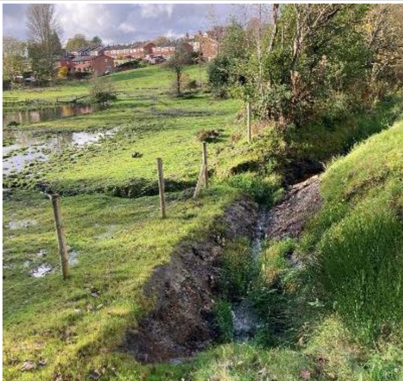
PLATE 6 EAST SITE - STREAM
