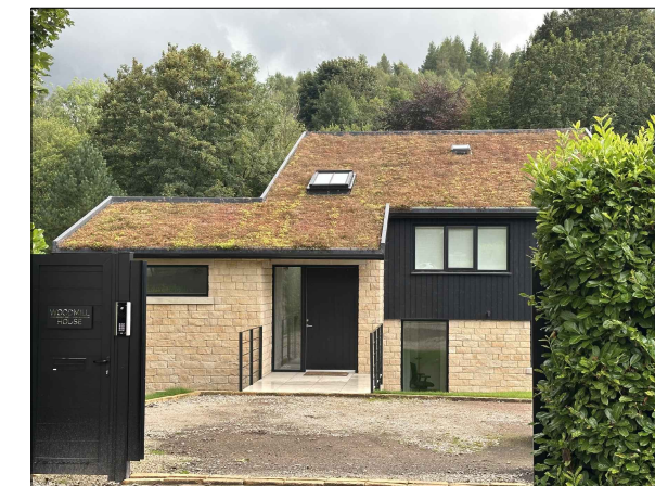
stonework with charred timber cladding (Saddleworth-Oldham)
