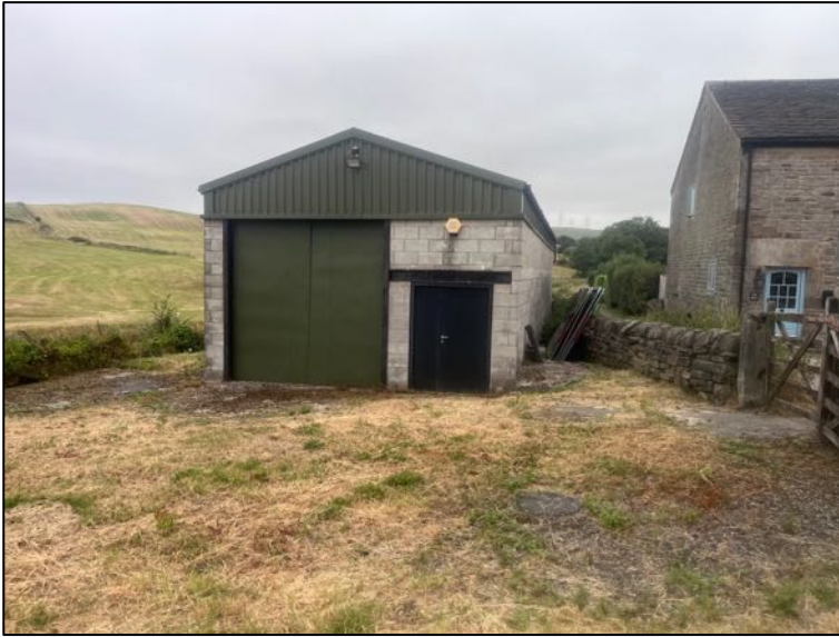
General view to the west across the site looking at the building
