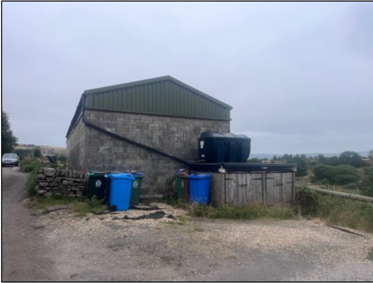
General view to the east of the eastern boundary with an above ground oil tank immediately adjacent and connecting to the site
