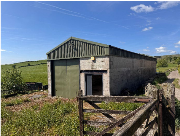
Existing Barn with existing green box cladding.
