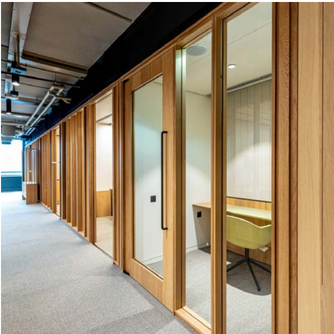
Examples of high quality timber framed glazing
