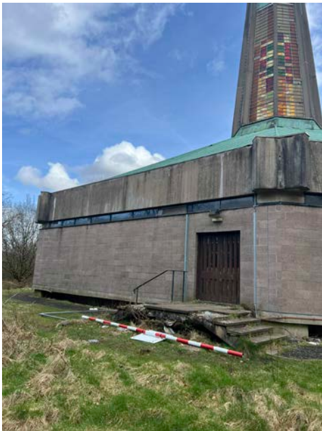
Rear steps to be retained and repaired
