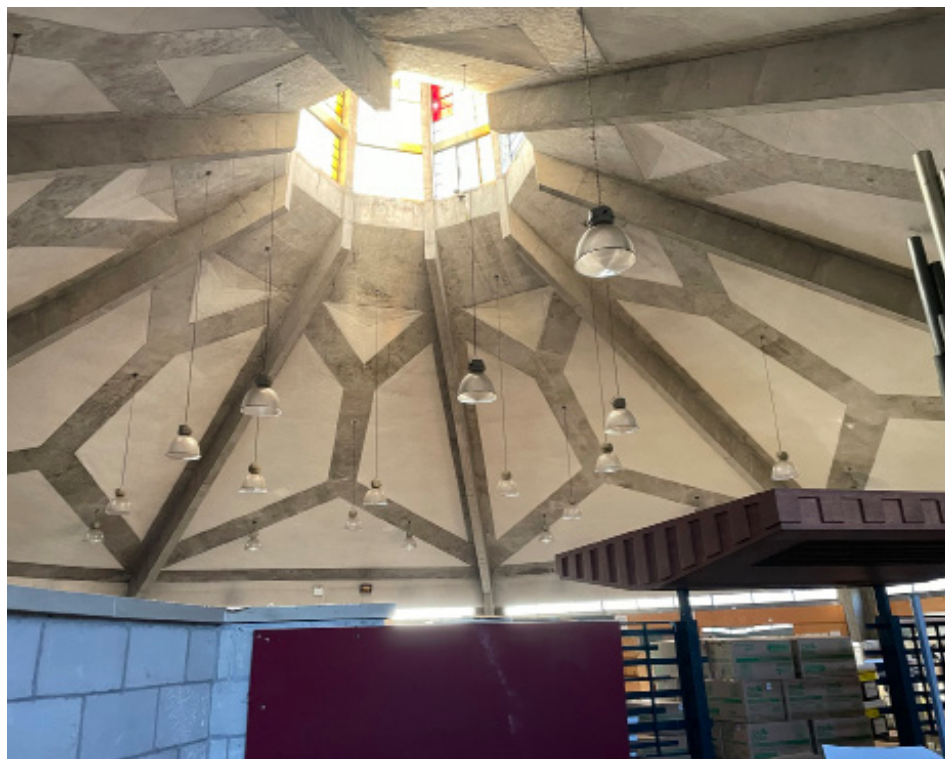
4 Internal view of octagonal roof structure.
