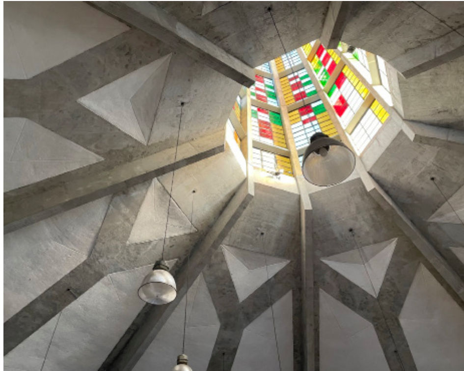
1 View looking up towards stain glass window.
