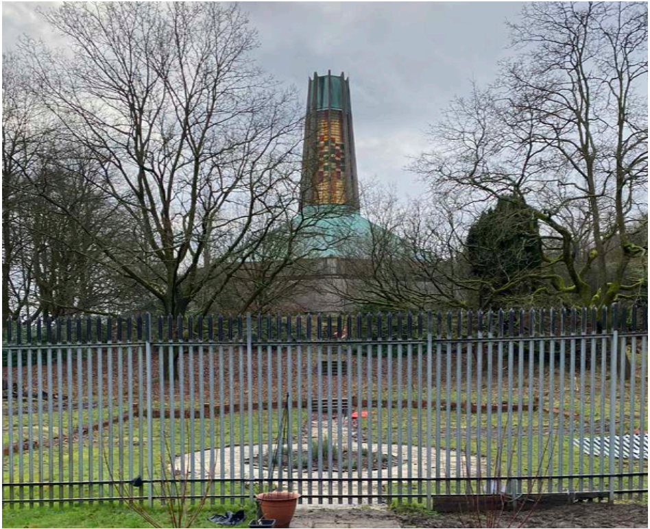
4 View towards the Chapel from Hopwood Hall grounds
