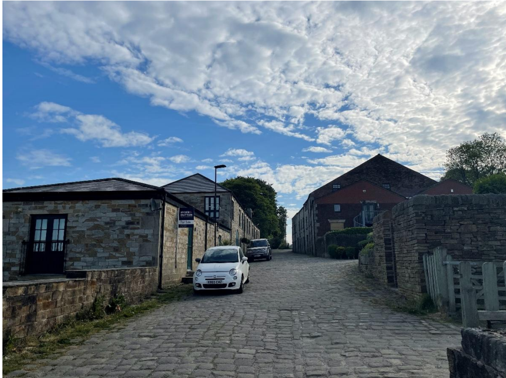
Figure 4.22: View looking north east along Clegg Hall Road within Clegg Village Conservation Area
