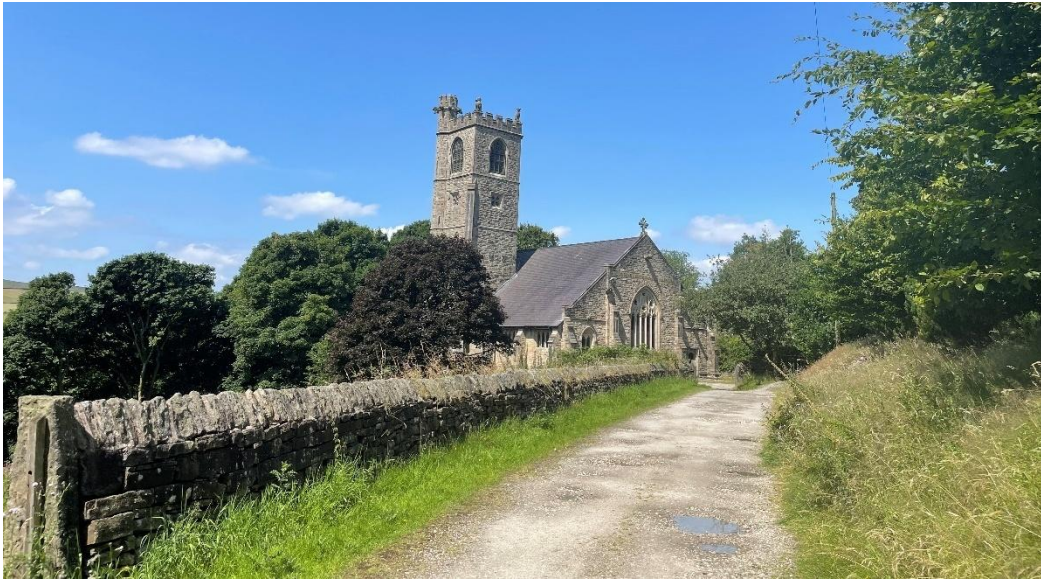
Figure 4.15: The Church of St Bartholomew, looking north. The rebuilt nave is out of scale with the Perpendicular style tower.
