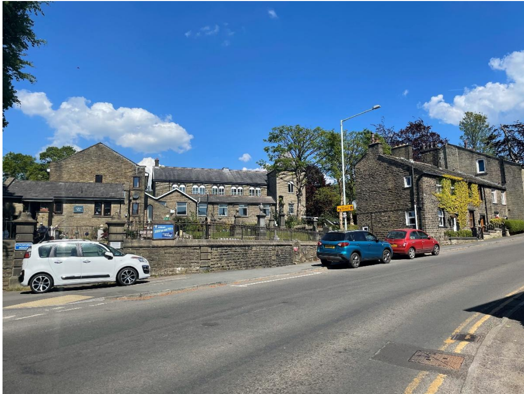
Figure 4.17: View looking north towards the Sion Baptist Chapel and other 19 th century buildings within the conservation area
