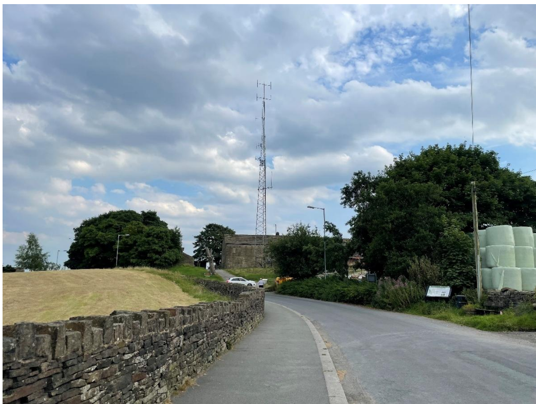
Figure 4.5: View looking south towards Brown Hill Farm, which lies at the southern end of the Conservation Area, and showing the large telephone antennae tower.
