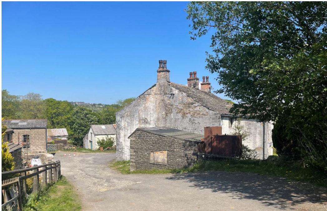
Figure 4.49: View looking northwards towards Fairwall Farmhouse and Barn, from the adjacent track, showing the rear and side elevation of the Farmhouse
