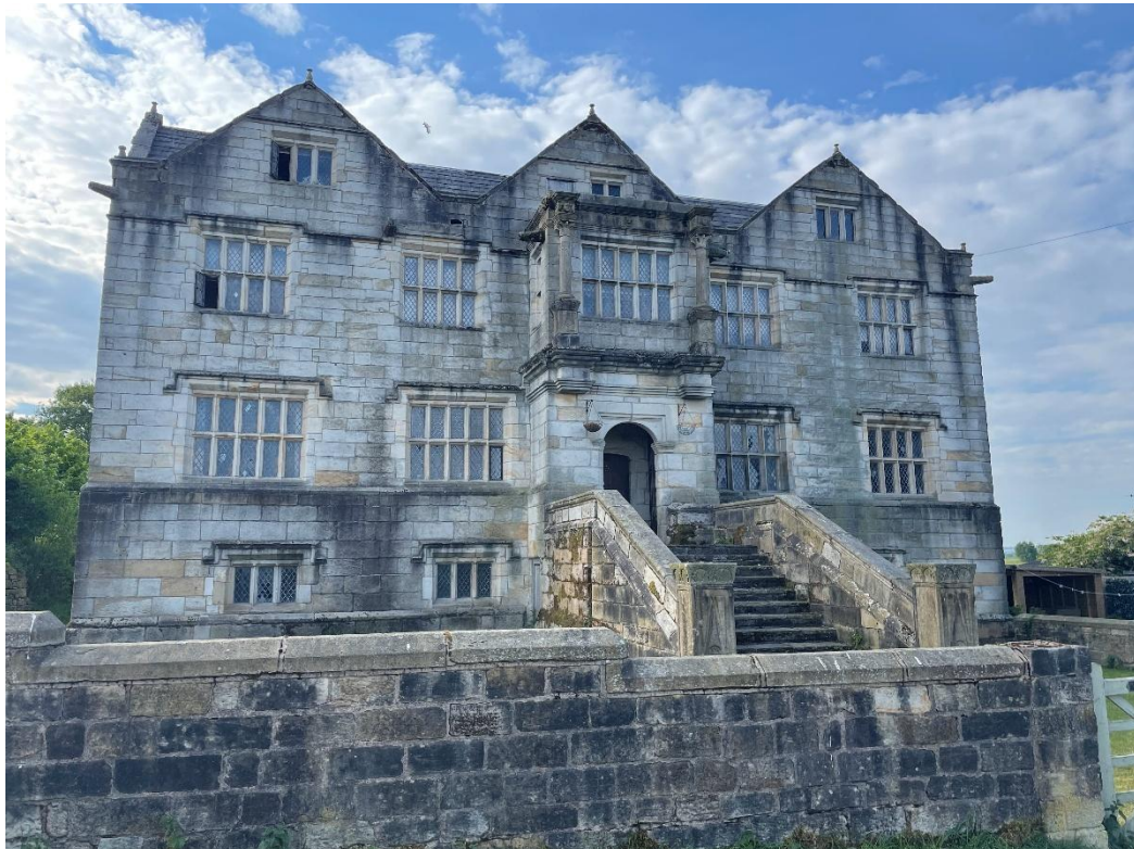
Figure 4.54: The principal elevation of Clegg Hall, looking south-east
