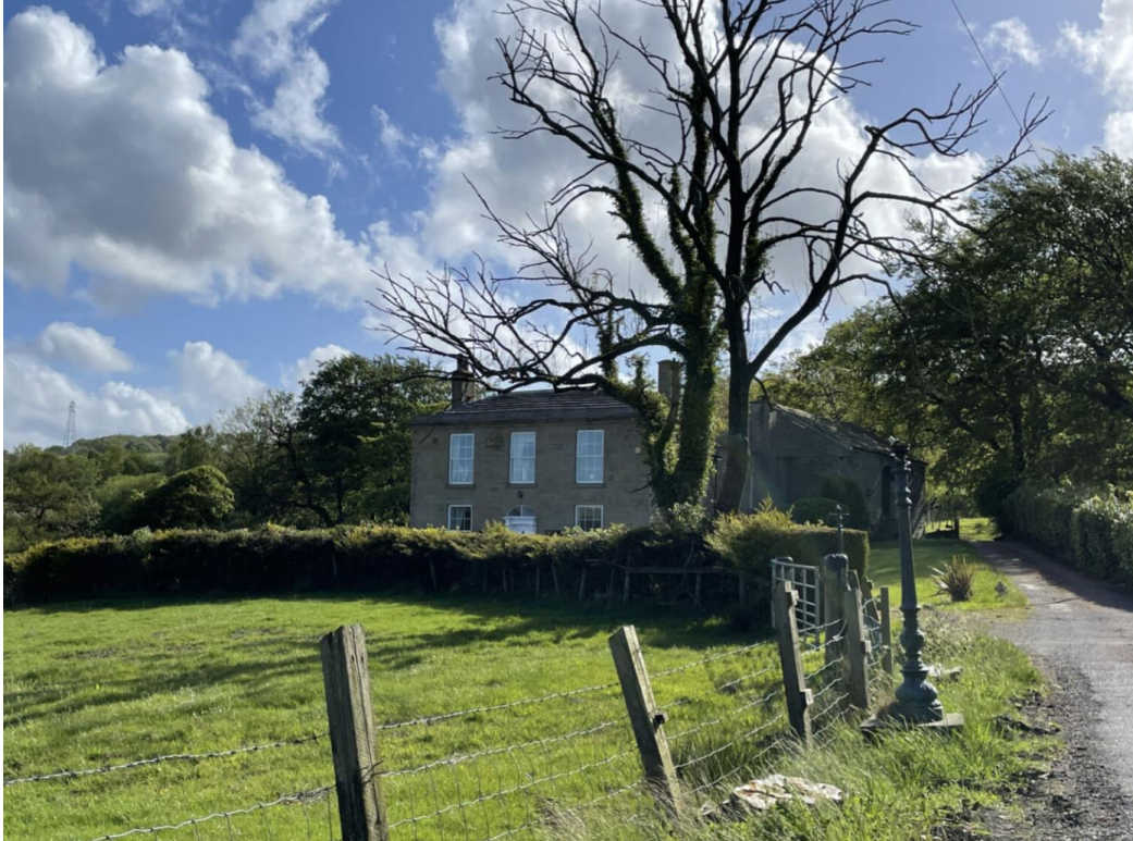
Figure 4.56: Spring Bank, looking west
