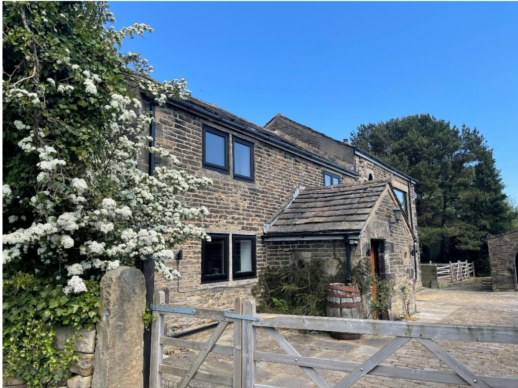
Figure 4.65: View looking north towards Harper Road House from Rooley Moor Road
