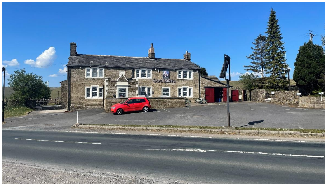
Figure 4.45: View of Owd Betts Public House from the south on Rochdale Road.
