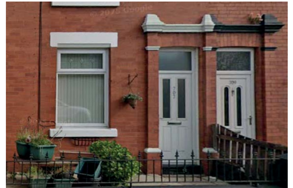
▲ Window detailing - Stone cills and lintels (Manchester Old Road)
