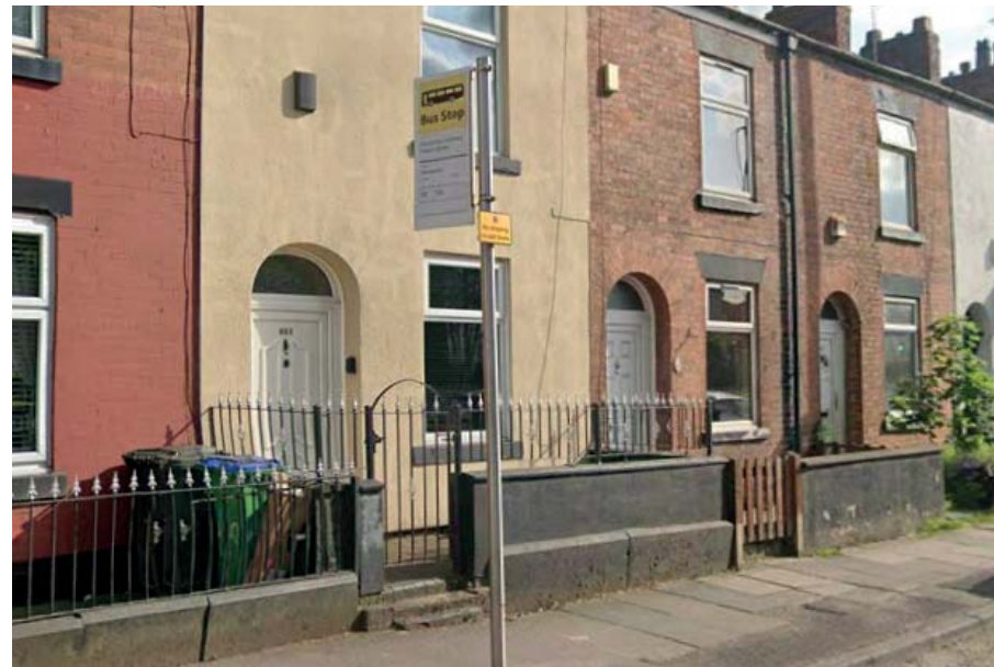
▲ Door detailing (Manchester Old Road)
