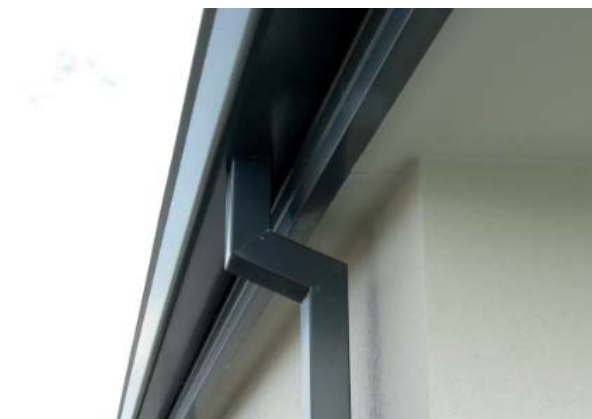
▲ uPVC rainwater goods
