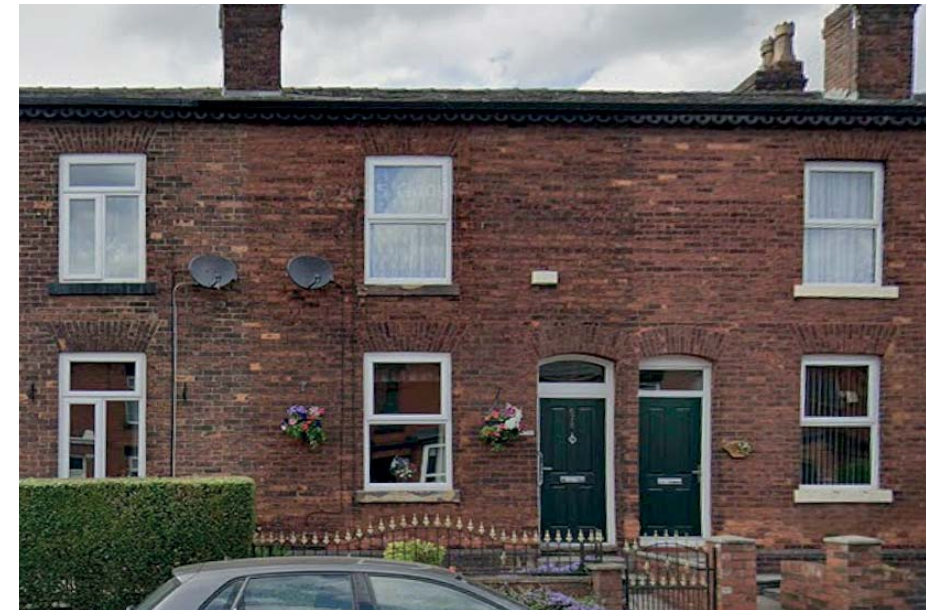
▲ Window proportions (Manchester Old Road)
