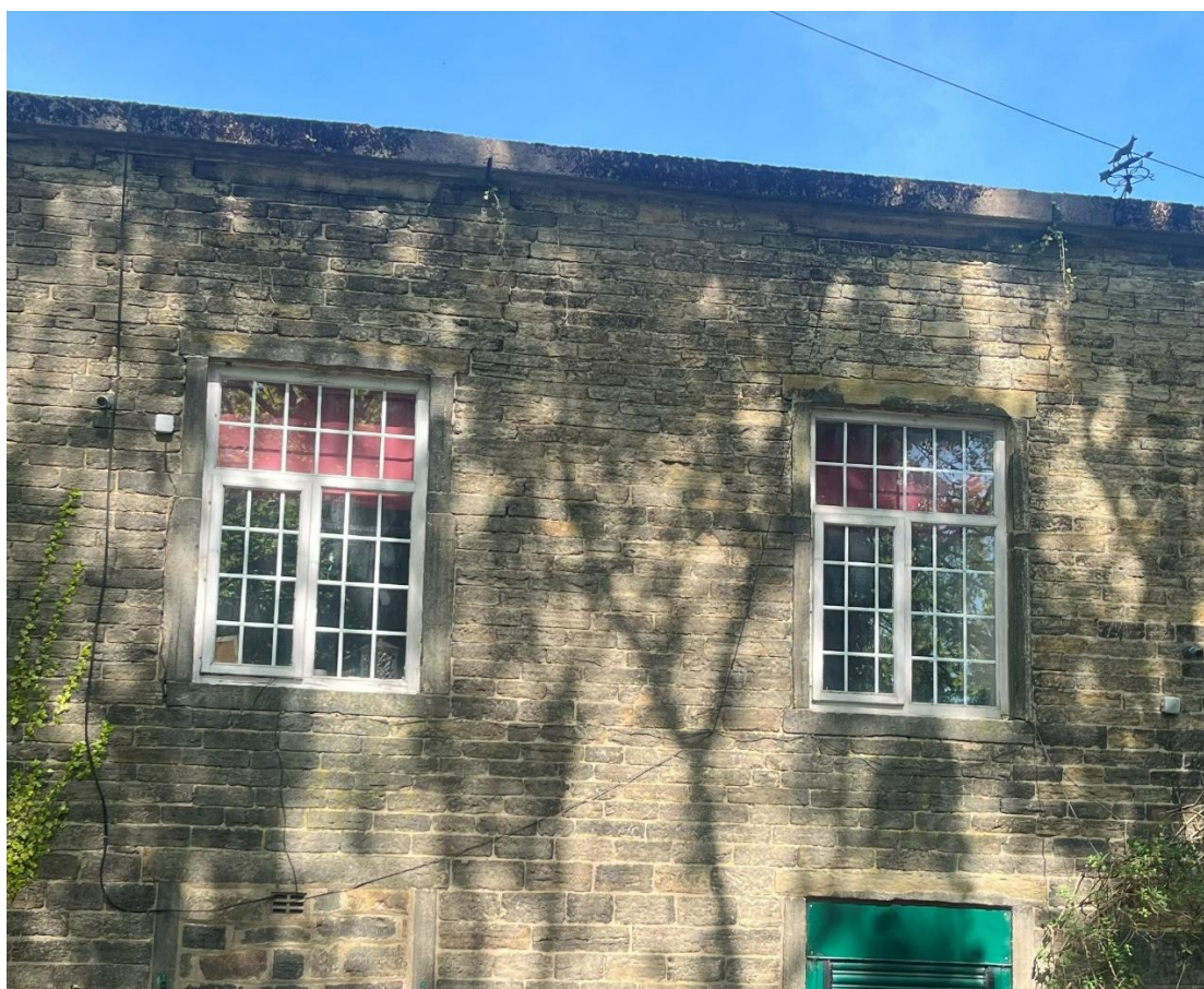
Figure 3. The front façade, note the arrangement of the window bays, the concrete copings and the possible window cills at eaves level. The window cills are also visible on the side elevation in similar bays.
