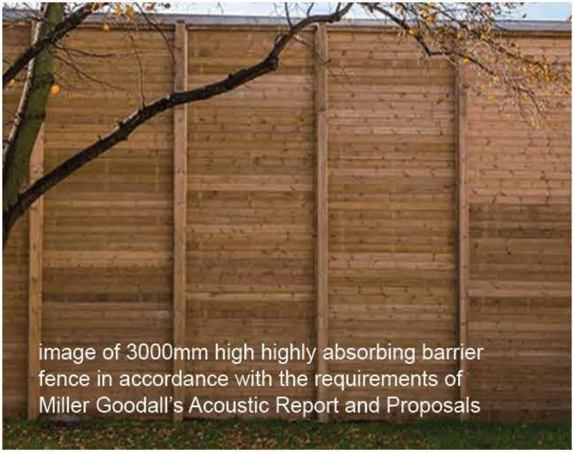
3000mm high fence: highly absorbing barrier
