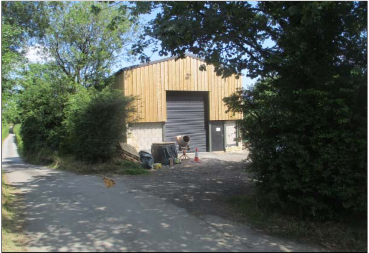
The agricultural shed northeast of the house
