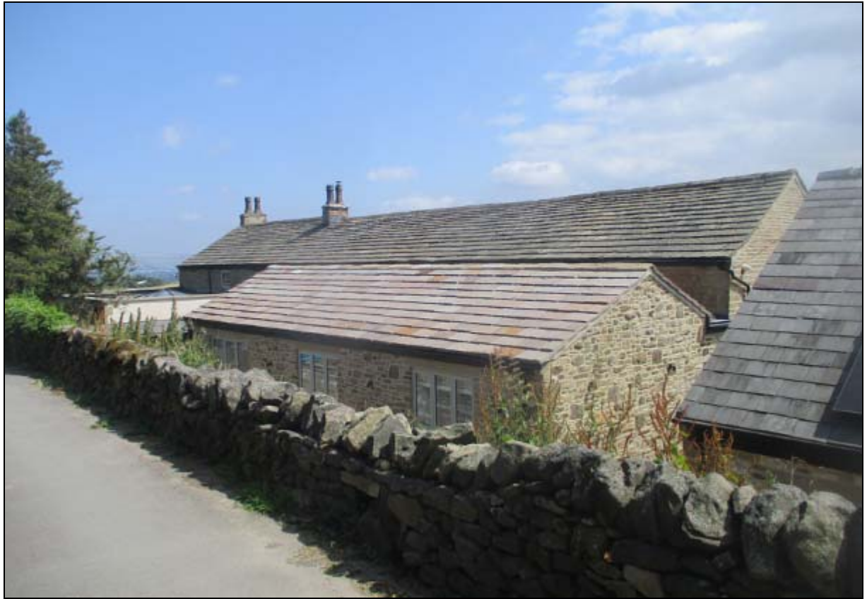
View of the rear from the track, showing prominent extensions to the barn
