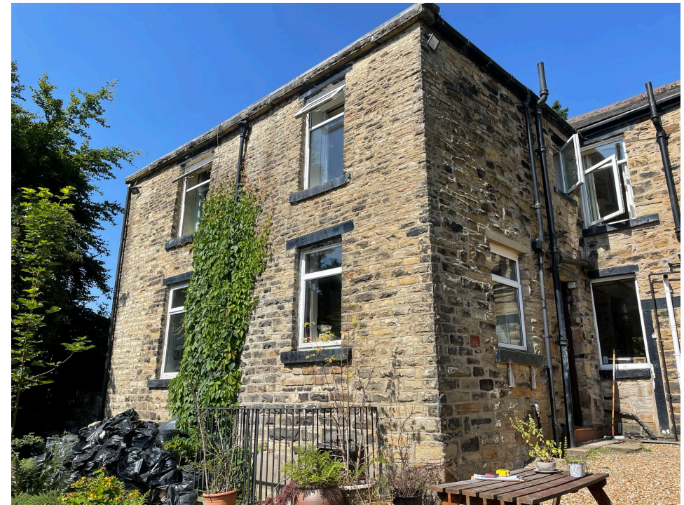
Fig.21 - Pitched faced stone to existing house
