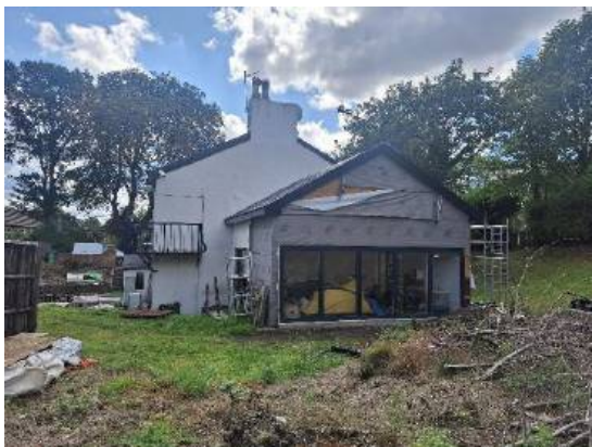
Photograph 5: Northern face of B1
