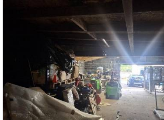
Photograph 8: Inside of B2
