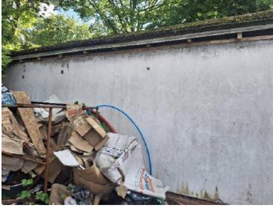
Photograph 7: Northern face of B2
