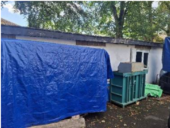
Photograph 9: Northern face of B3
