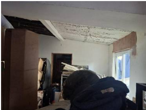
Photograph 11: Inside of B3
