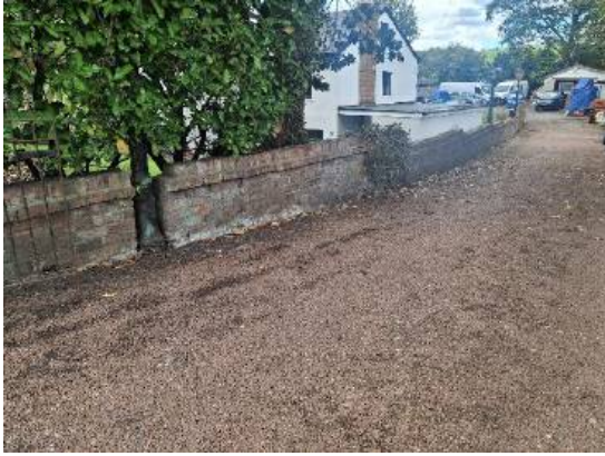
Photograph 19: Wall along hardstanding entrance to site
