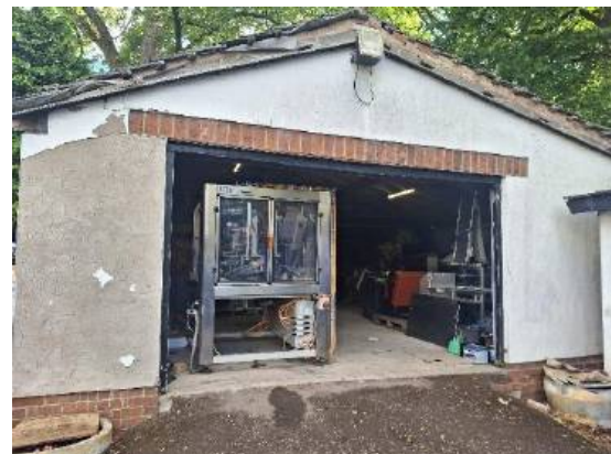
Photograph 6: Western face of B2
