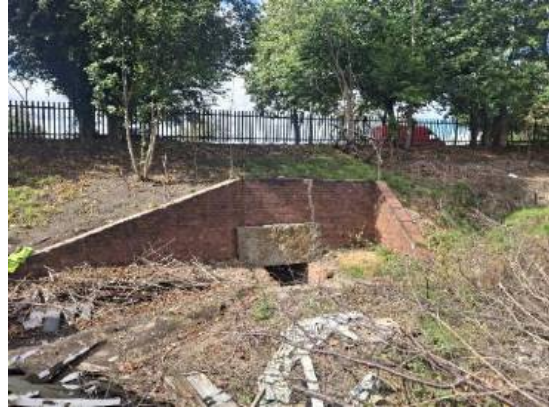
Photograph 20: Wall structure northwest of B1
