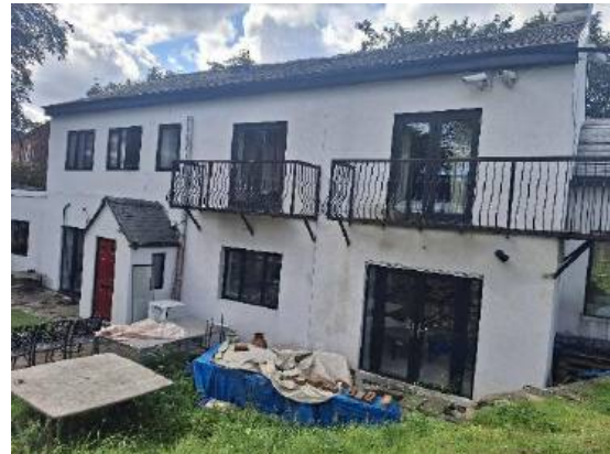
Photograph 2: Eastern face of B1
