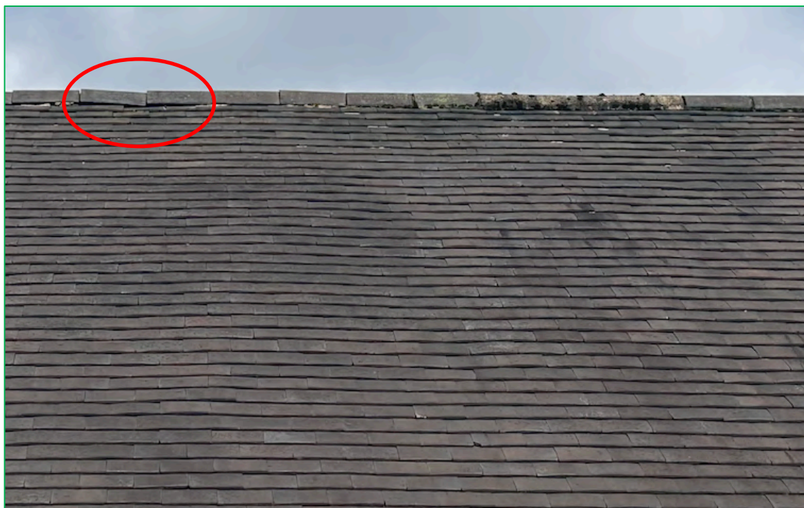
Showing well-sealed tiles on the south elevation with a gap under the ridge tiles
