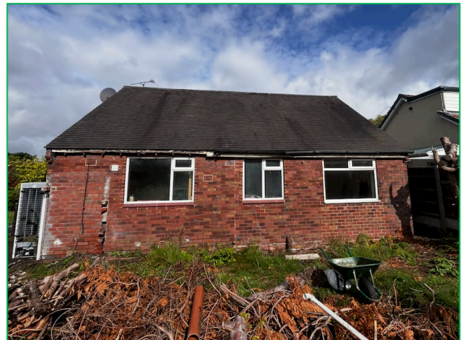
The rear (south) elevation of the house
