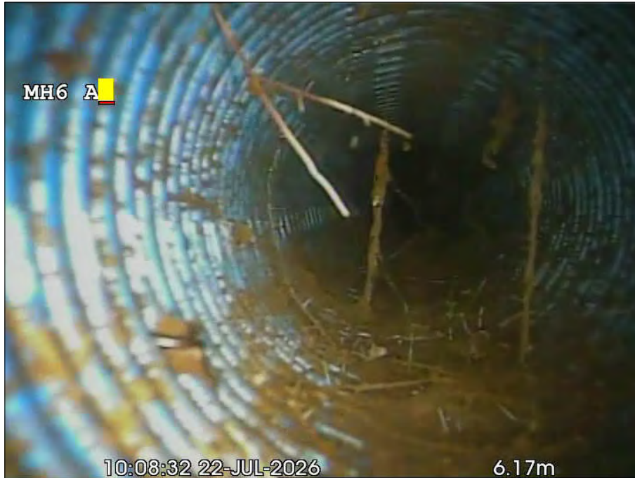
Photo: 28_7a, 00:00:00 6m, Fine Roots, Start
