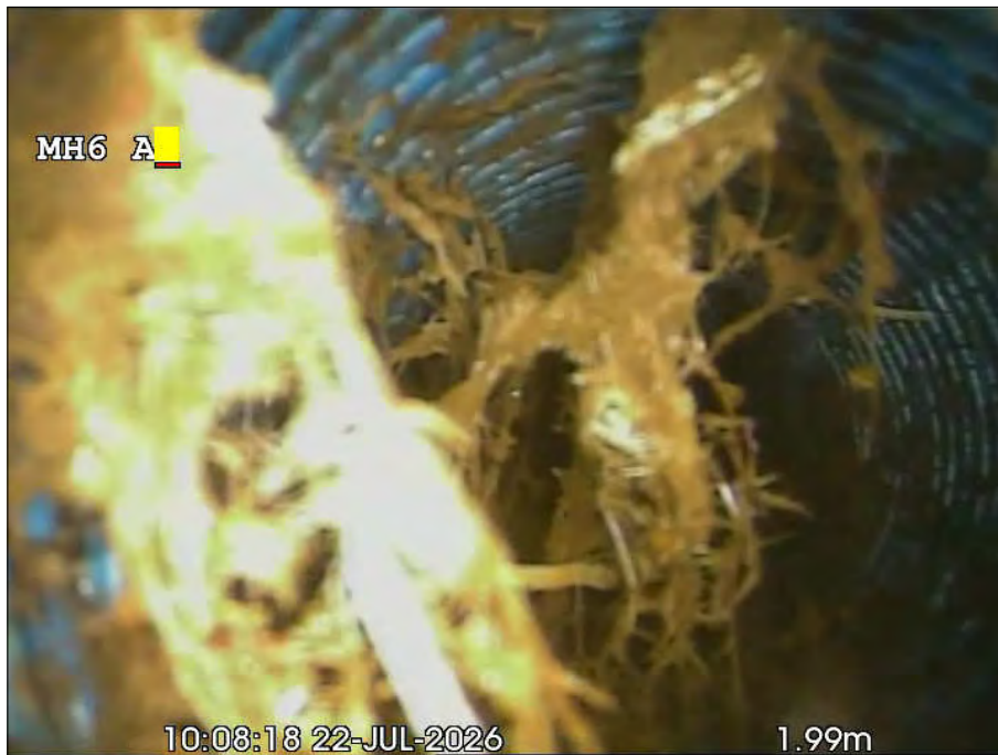
Photo: 28_5a, 00:00:00 1.2m, Mass Roots 10 % cross-sectional area loss, Start
