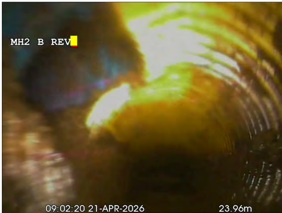
Photo: 32_11a, 00:00:00 24m, Connection, at 09 o'clock, dia 80 mm
