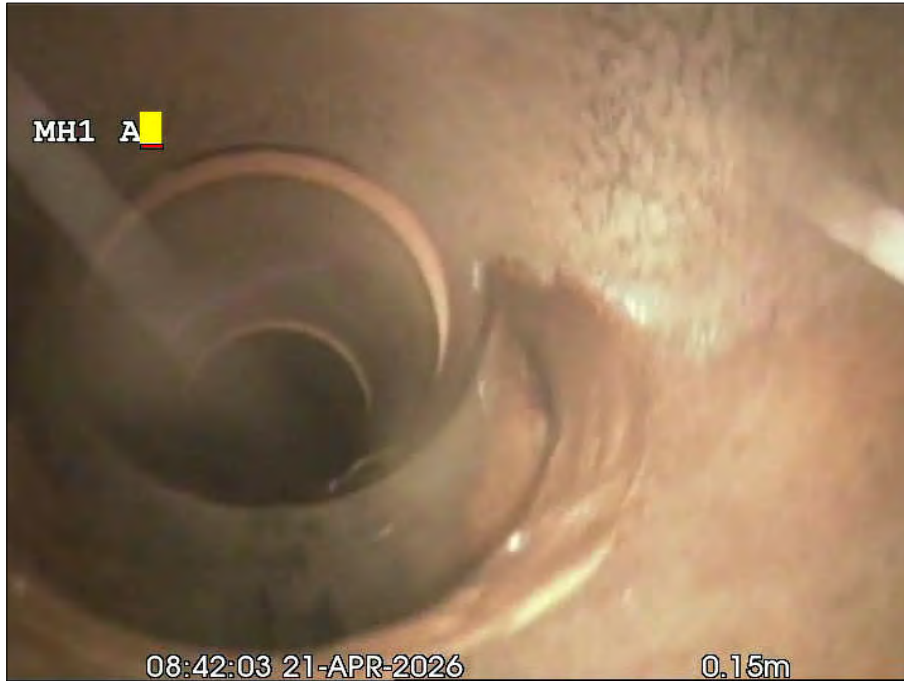
Photo: 317_4a, 00:00:00 0.1m, Junction at 06 o'clock, dia 150 mm
