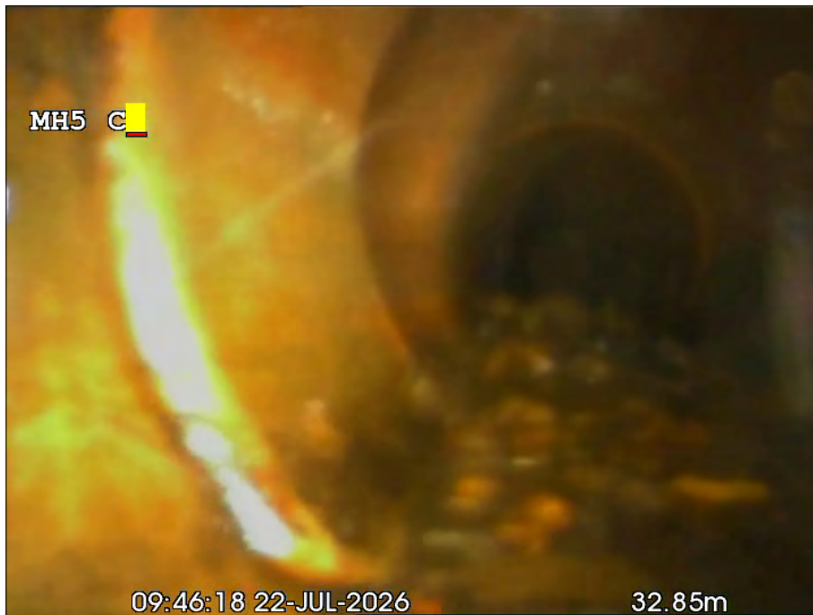
Photo: 24_14a, 00:00:00 33m, Junction at 09 o'clock, dia 150 mm
