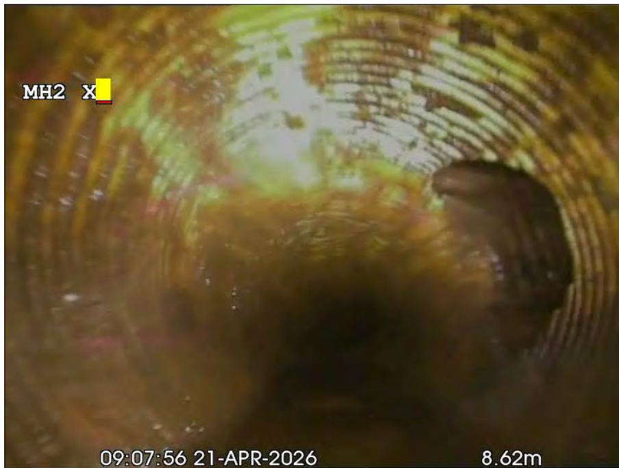
Photo: 304_7a, 00:00:00 8.8m, Junction at 03 o'clock, dia 100 mm
