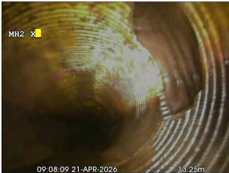
Photo: 308_10a, 00:00:00 13.3m, Junction at 03 o'clock, dia 100 mm
