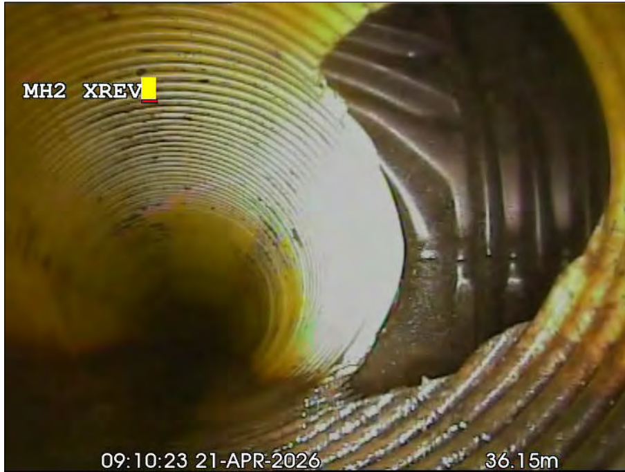
Photo: 34_15a, 00:00:00 36.2m, Junction at 03 o'clock, dia 100 mm
