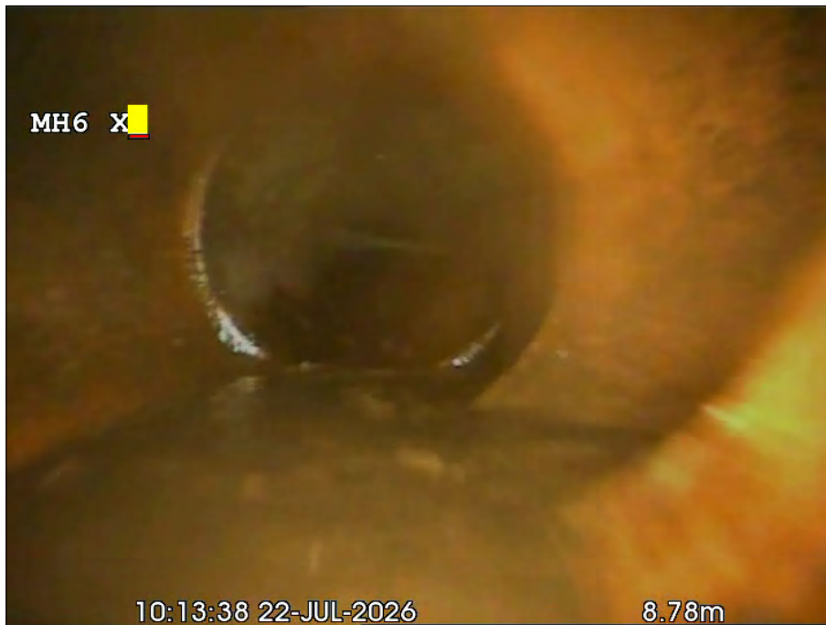
Photo: 30_5a, 00:00:00 8.7m, Junction at 03 o'clock, dia 100 mm
