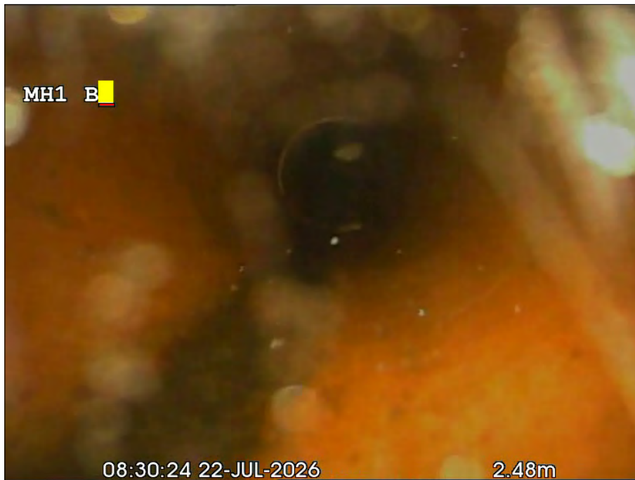
Photo: 233_7a, 00:00:00 2.5m, Debris, 10 % cross-sectional area loss, Finish
