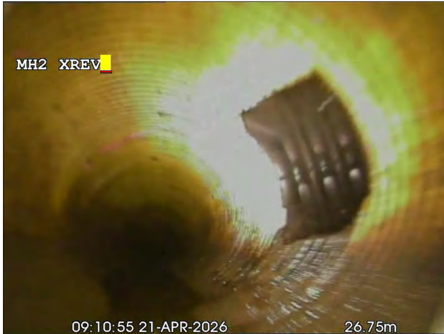
Photo: 34_13a, 00:00:00 26.8m, Junction at 03 o'clock, dia 100 mm
