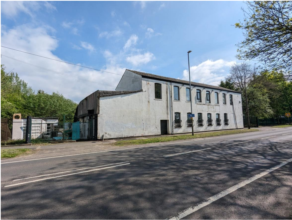
Figure 1: Existing principal elevation and rear/side return, viewed from Heywood Old Road.
