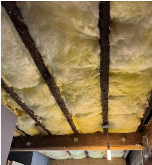
Acoustic Mineral wool in use - Ceilings / Floors
