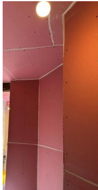
Second layer – Fireboard for protected route Intumescent / Acoustic sealant in use
