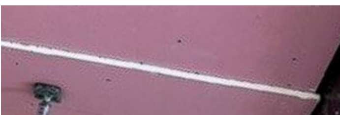
First Floor ceiling – double boarding
