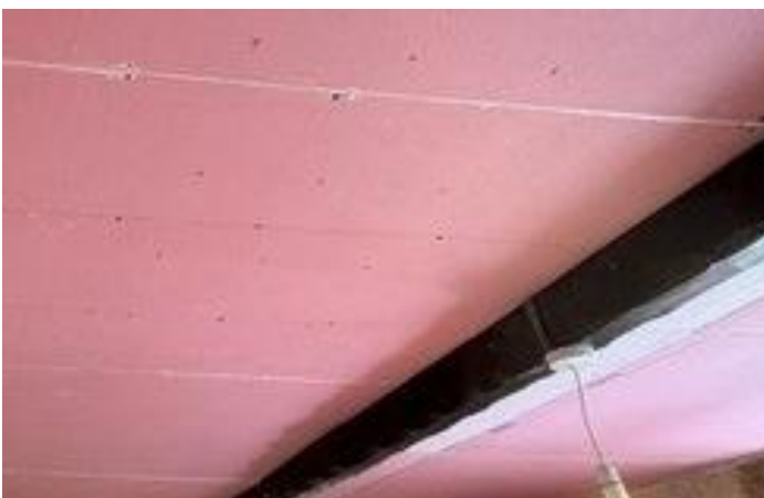
Ground floor Hallway - First layer sound board
