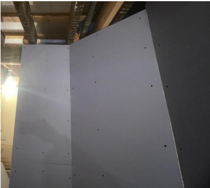
Ground floor Hallway - First layer sound board
