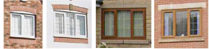
Window heads and cill details vary from red soldier bricks to stone in different heights, widths and styles, whether it be arched or linear.
