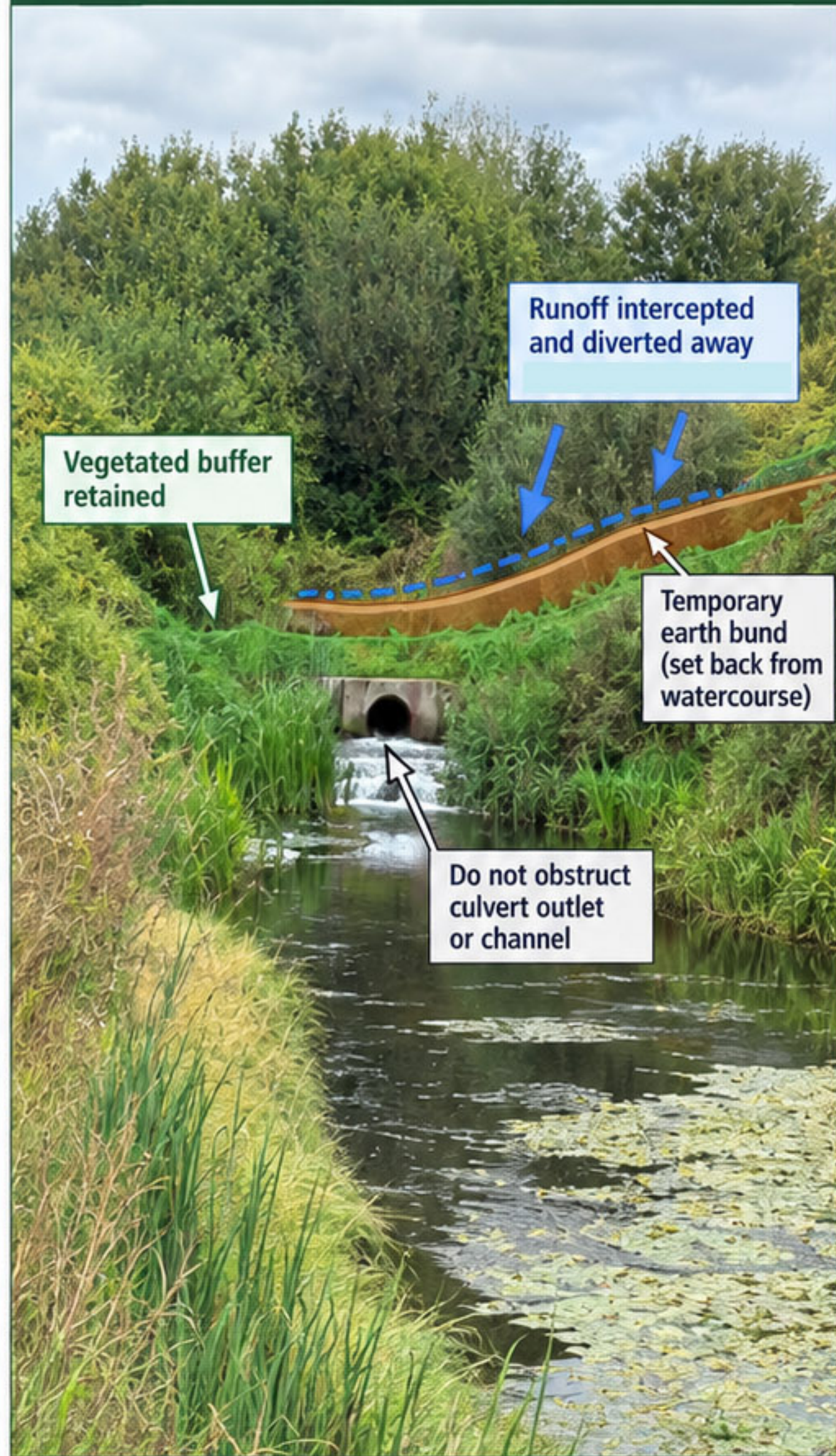
B. Downstream view towards outlet (view downstream)
