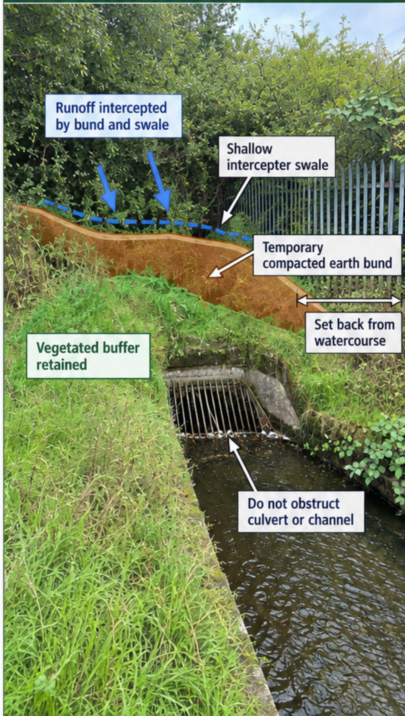
A. Culvert inlet and channel edge (view upstream)
