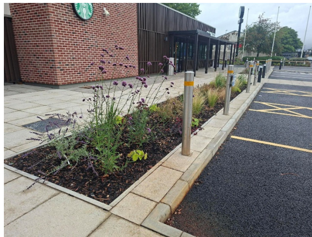
Image 5: Thin cover of bark over 230mm of brown sandy clay topsoil
