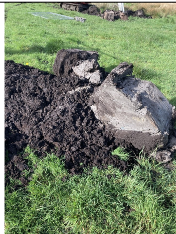
Trial Pit 115/ Soakaway 103 Spoil
