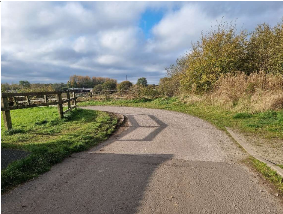
Photo 02 – Culvert bridge – west approach
