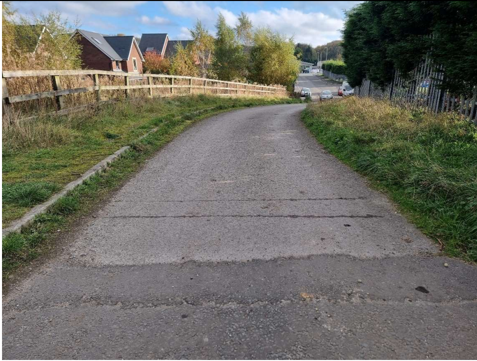
Photo 01 – Culvert bridge – east approach
