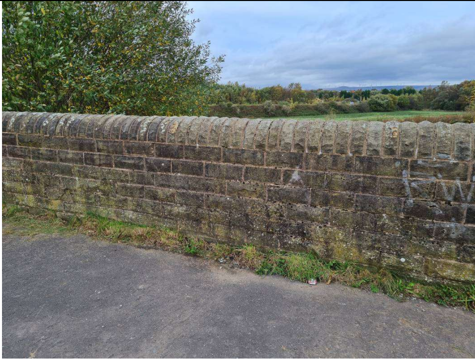
Photo 05 – Culvert bridge – north parapet internal
