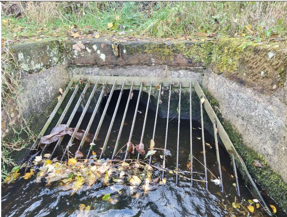
Photo 10 – Buried culvert pipe – inlet
