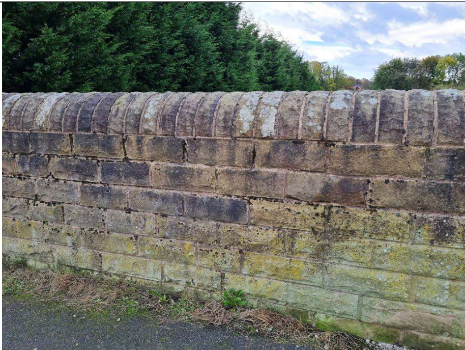
Photo 06 – Culvert bridge – south parapet internal
