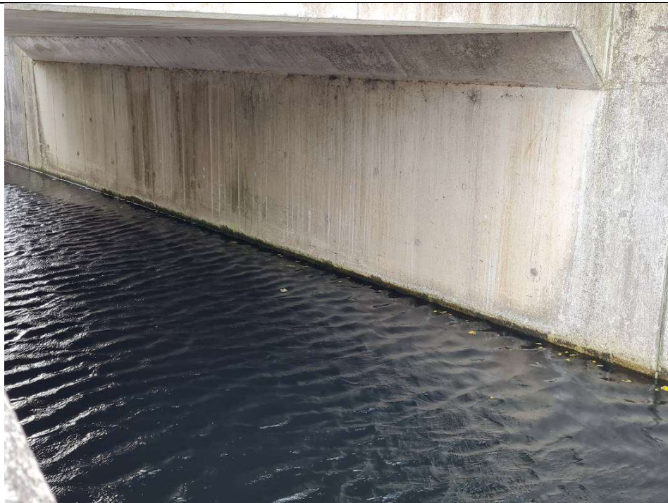
Photo 08 – Culvert bridge – west abutment wall
