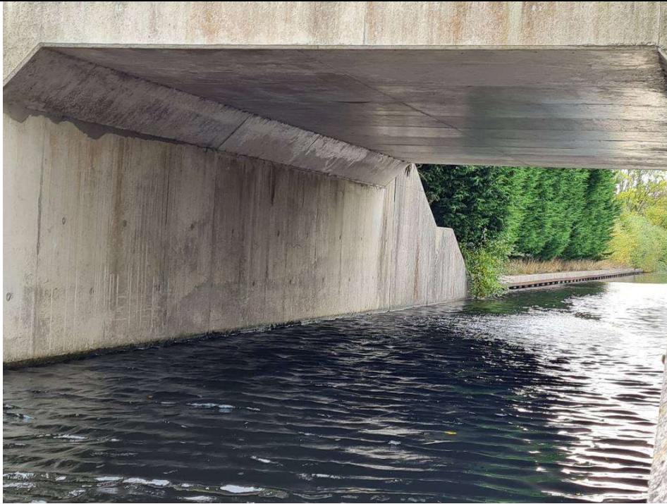
Photo 09 – Culvert bridge – deck soffit
