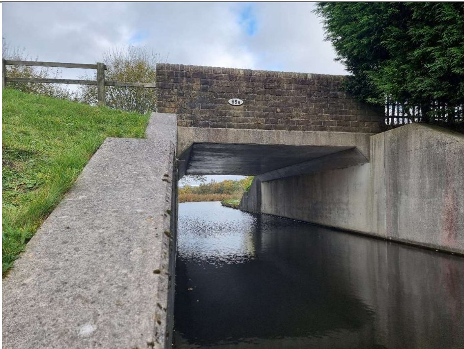
Photo 04 – Culvert bridge – south elevation
