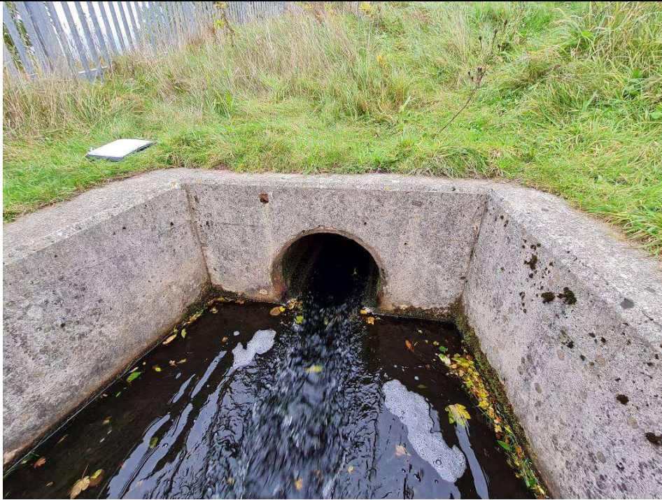
Photo 11 – Buried culvert pipe – outlet
