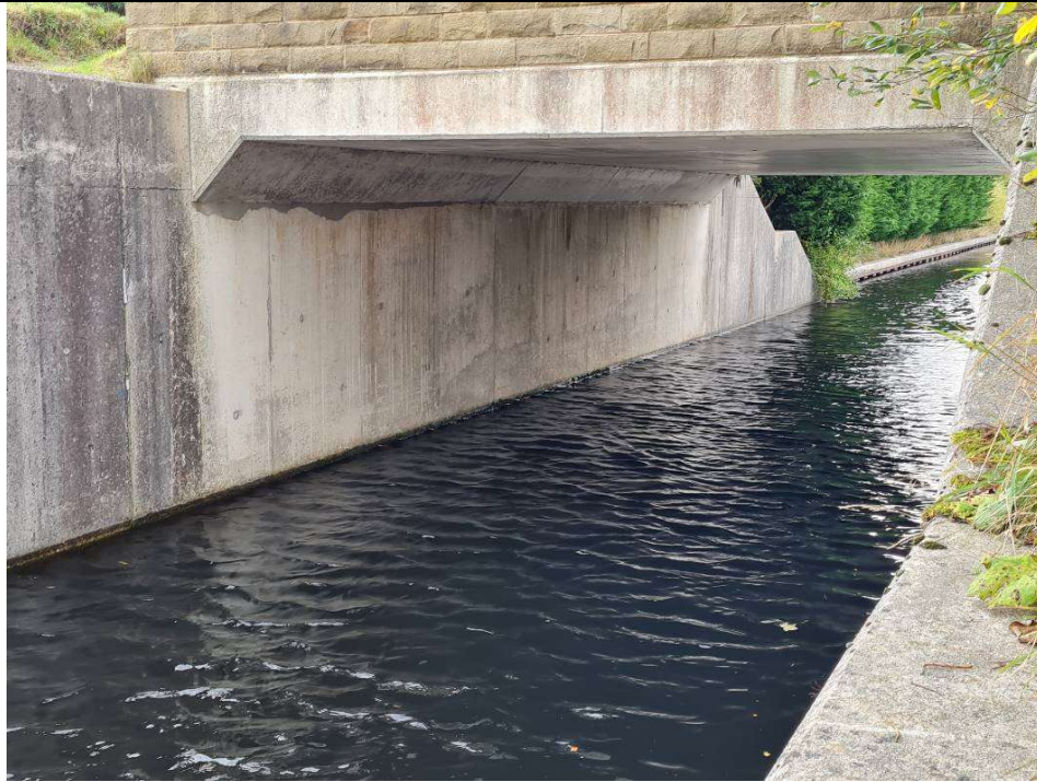
Photo 07 – Culvert bridge – east abutment wall
