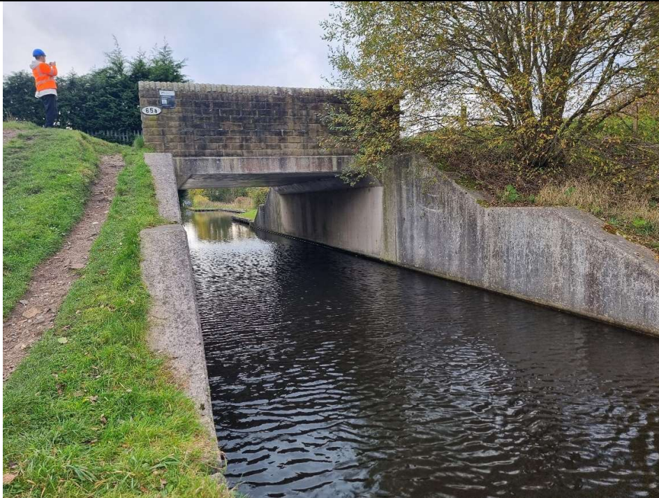
Photo 03 – Culvert bridge – north elevation
