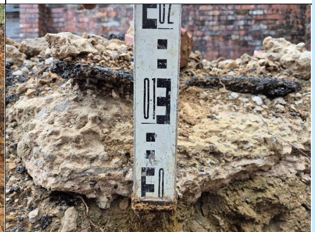
P8: TP2 asphalt and concrete surface layers
