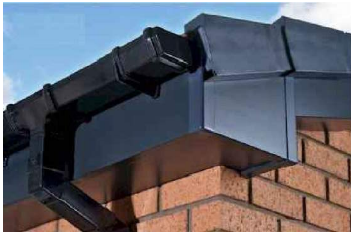
(B) Eaves Slate grey eaves boards (RAL7015)
