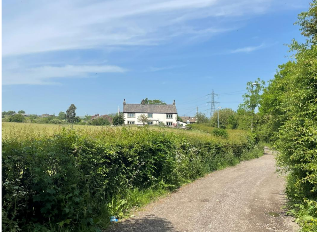
Figure 4.11: View of Hollin Hall Cottage from the south on Jowkin Lane
