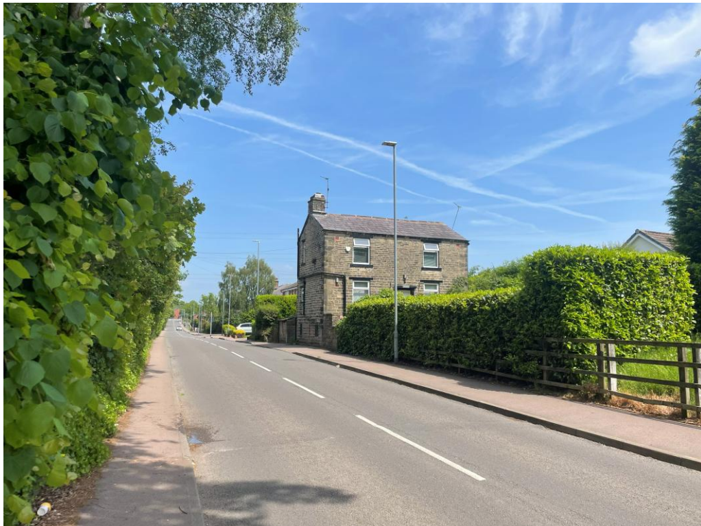
Figure 4.7: View of 36-38 Norden Road from the south west on Norden Road
