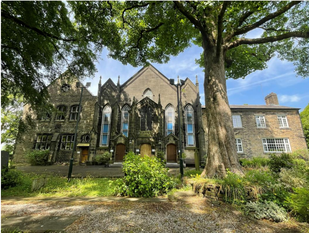
Figure 4.2: View of the Bamford United Reformed Church and Bamford Chapel from the south within the churchyard
