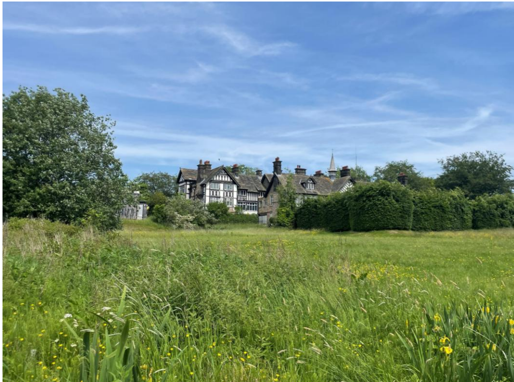
Figure 4.16: View of Scott House from the south west
