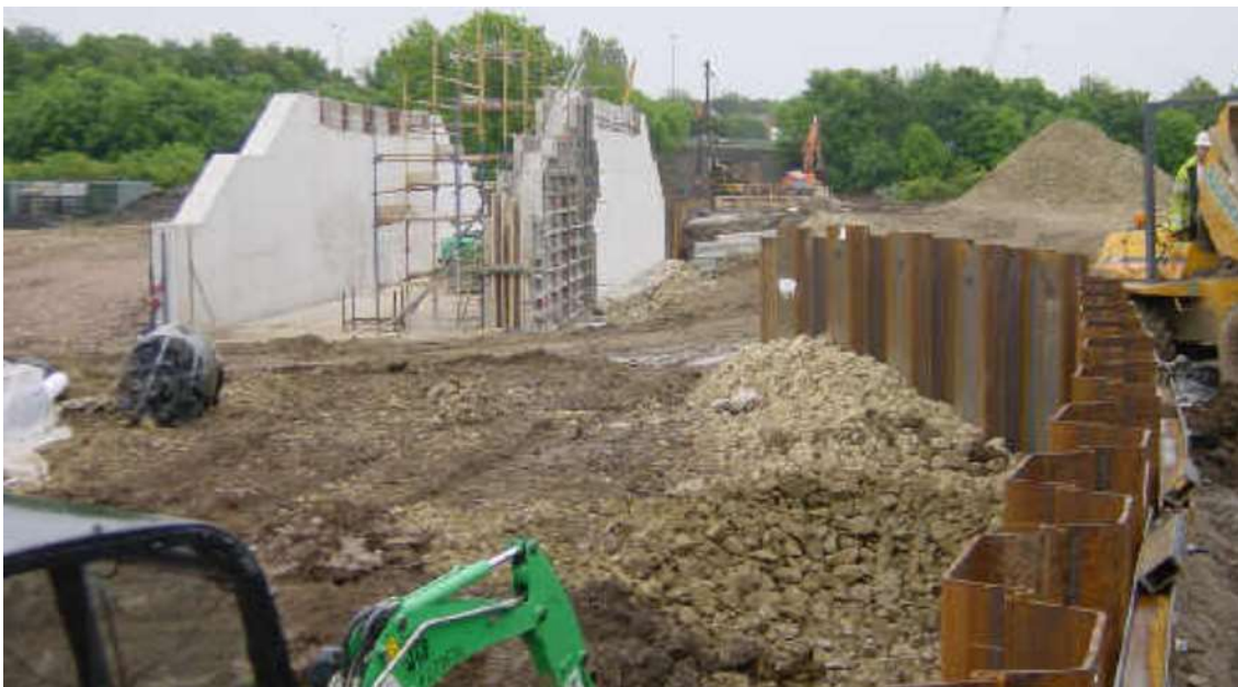
Figure 9 – New Bridge Construction Looking South Towards the M62 Circa 2002 2
