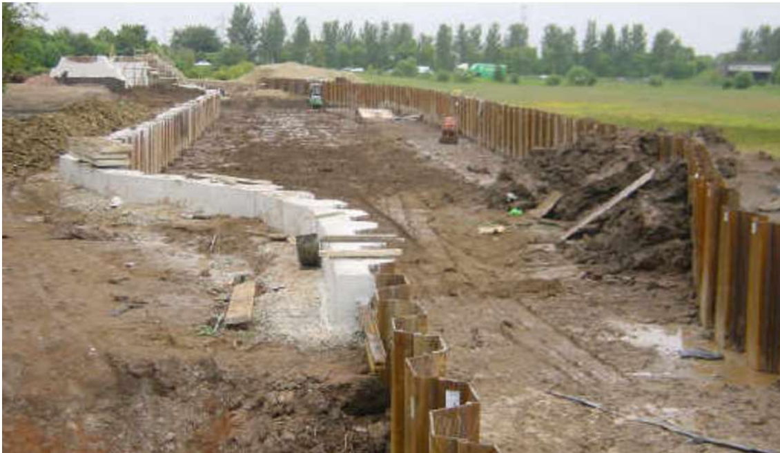
Figure 8 – Looking South From Old lock 53 Towards the New Bridge Circa 2002 2
